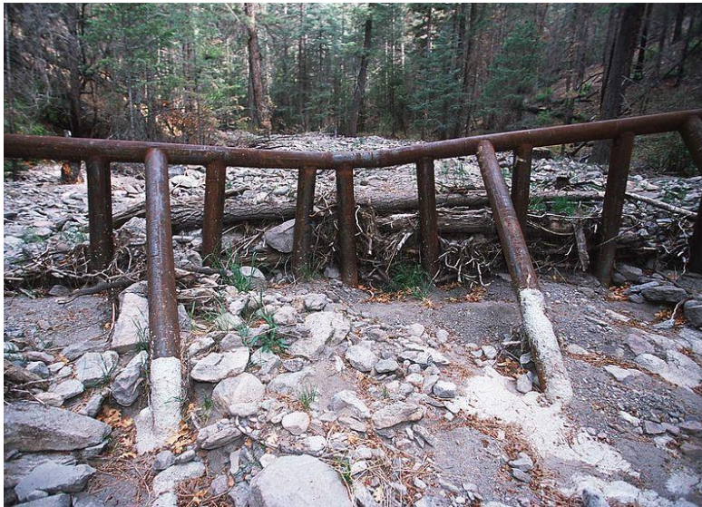
Figure 6. Example #1 of an Upstream Debris Catcher
