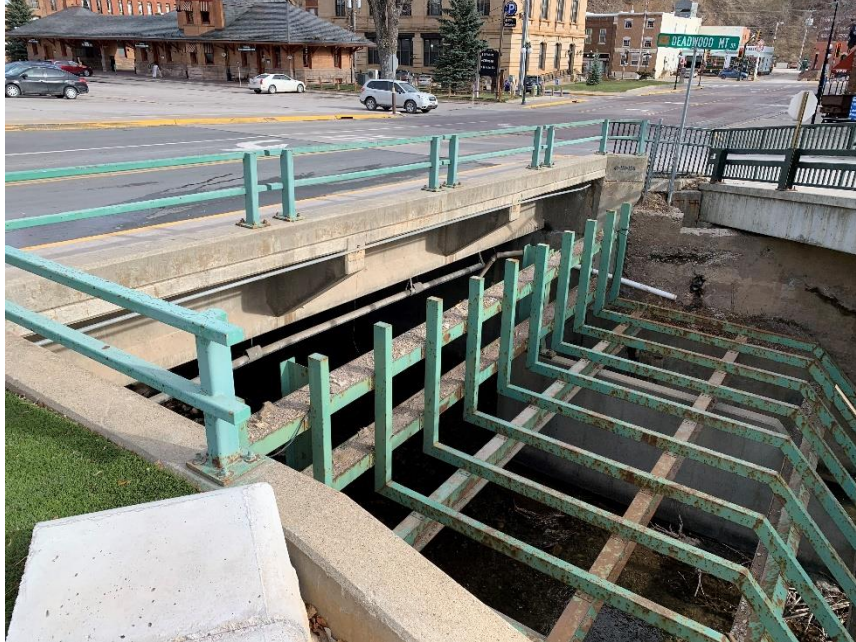
Figure 4. Existing Debris Catcher Secured to Box Inlet Adjacent to Pine Street
