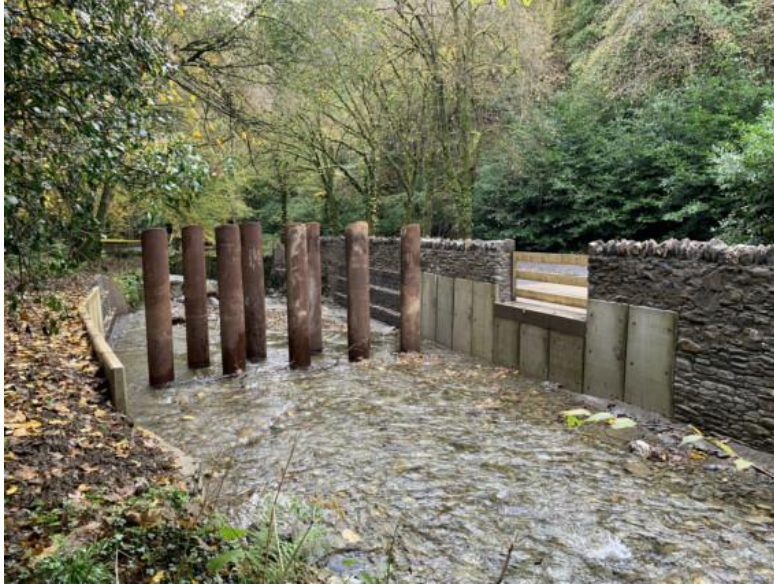
Figure 6. Example #1 of an Upstream Debris Catcher
