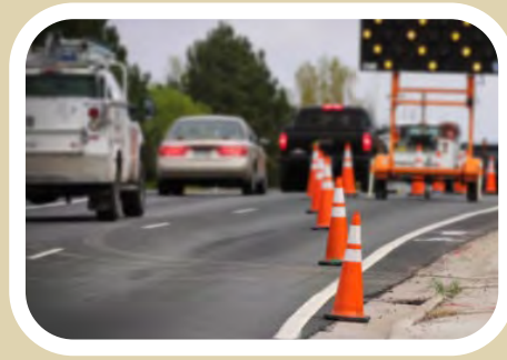
Traffic Accommodating During Construction
