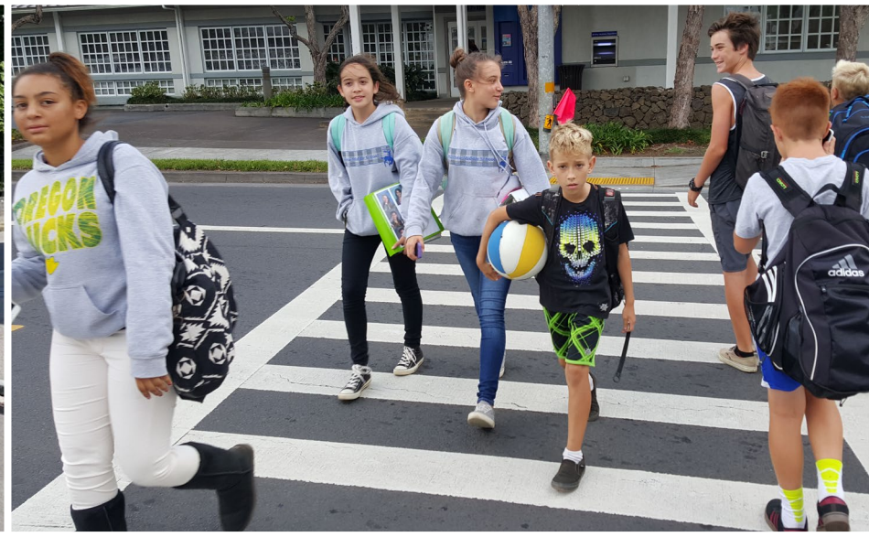
Ladder Style High Visibility Crosswalk Marking
