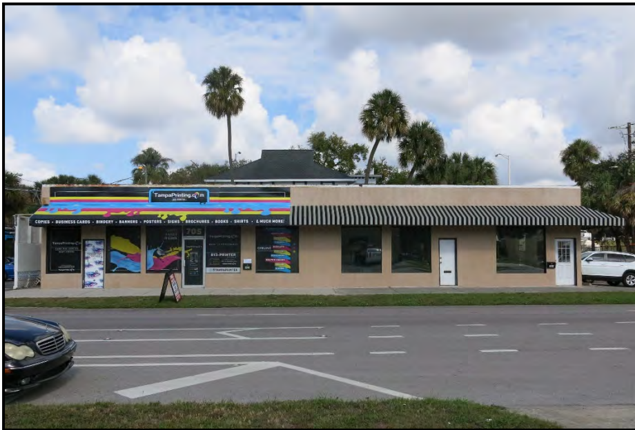
Photo 5.22. 701 W Platt St (8HI14821), looking north.
