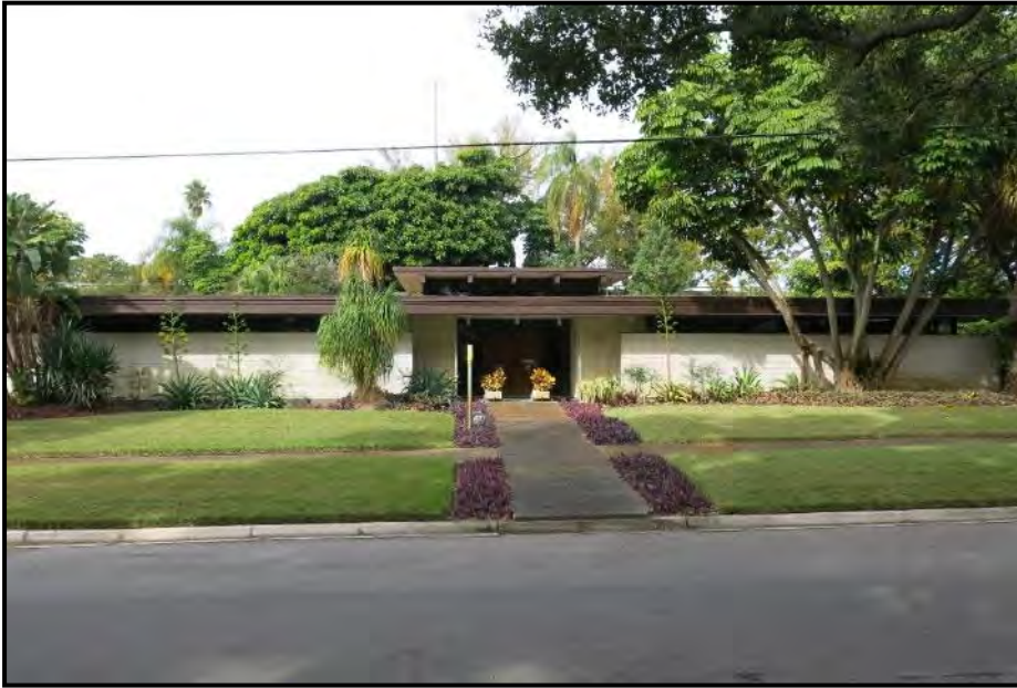
Photo 5.6. 3501 S Drexel Avenue (8HI14745), looking northwest.
