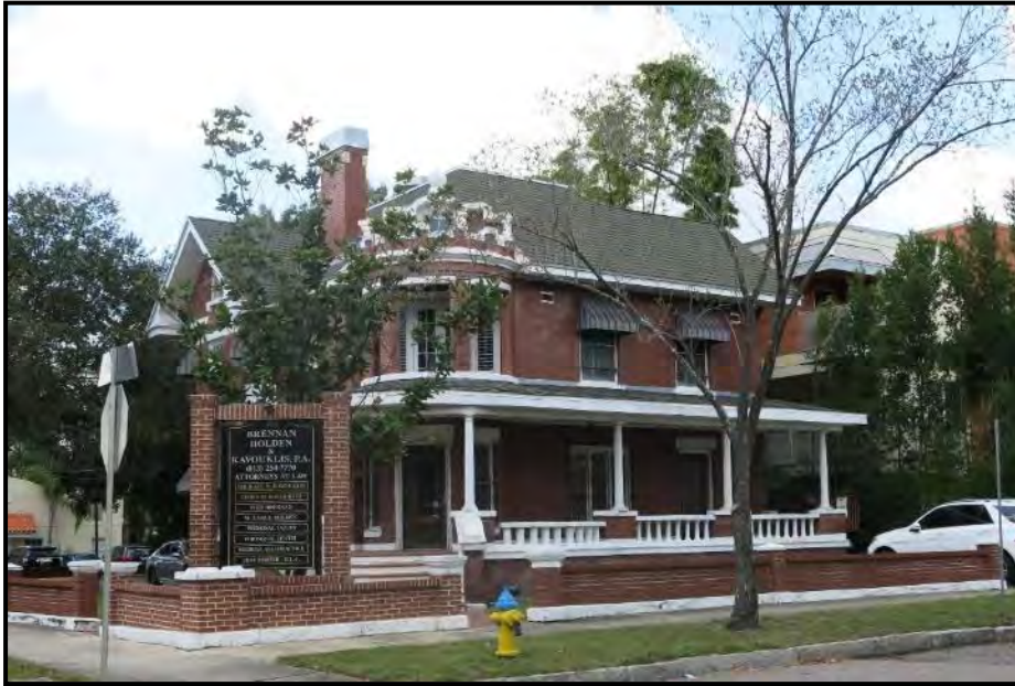
Photo 5.34. 115 S Newport Ave (8HI01439), looking northwest.
