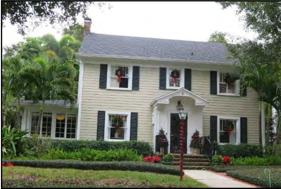
Photo 5.30. 2406 W Prospect Rd (8HI07211), looking southeast.
