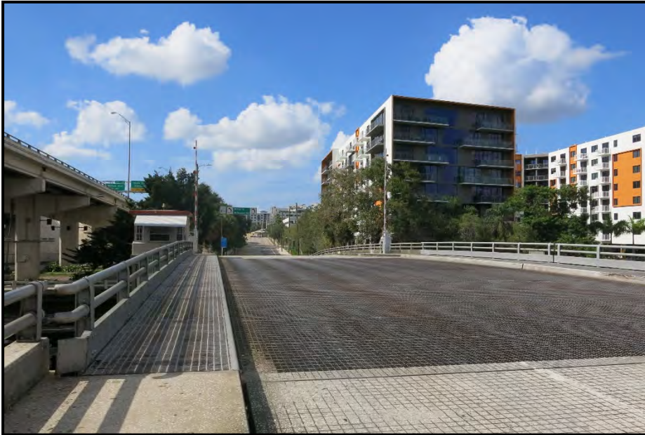
Photo 5.16. Brorein Bridge; FDOT Bridge No. 105501 (8HI11540), looking northwest.
