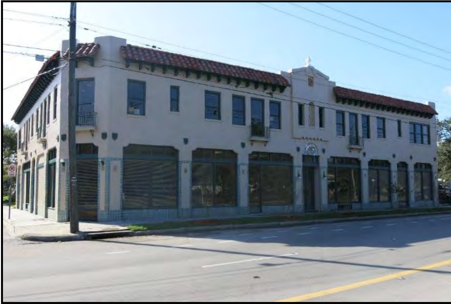
Photo 5.32. 1200 Platt St (8HI01318), looking southwest.
