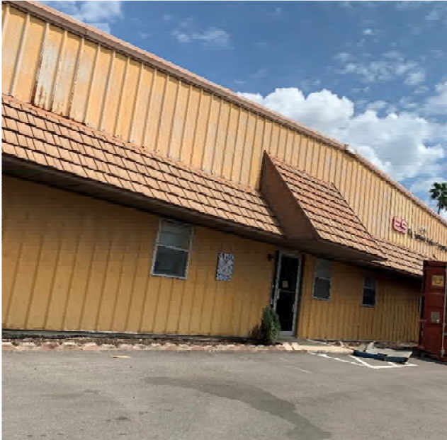
Site 19 - Currently Abandoned Property
