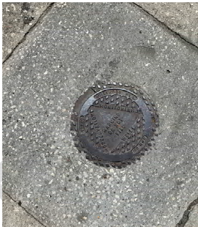
Site 71 - Currently Boca Tampa Restaurant Monitoring well in site parking lot
