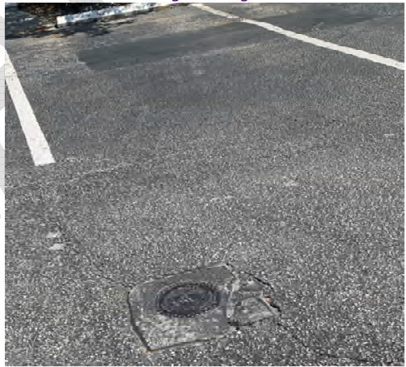
Site – 68 Ciccio Water Restaurant Monitoring well in site parking lot (facing east)
