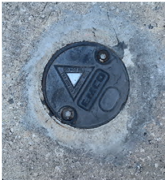
Site 71 - Currently Boca Tampa Restaurant Monitoring well in site parking lot
