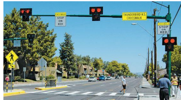
Rectangular Rapid-Flashing Beacon (RRFB)
