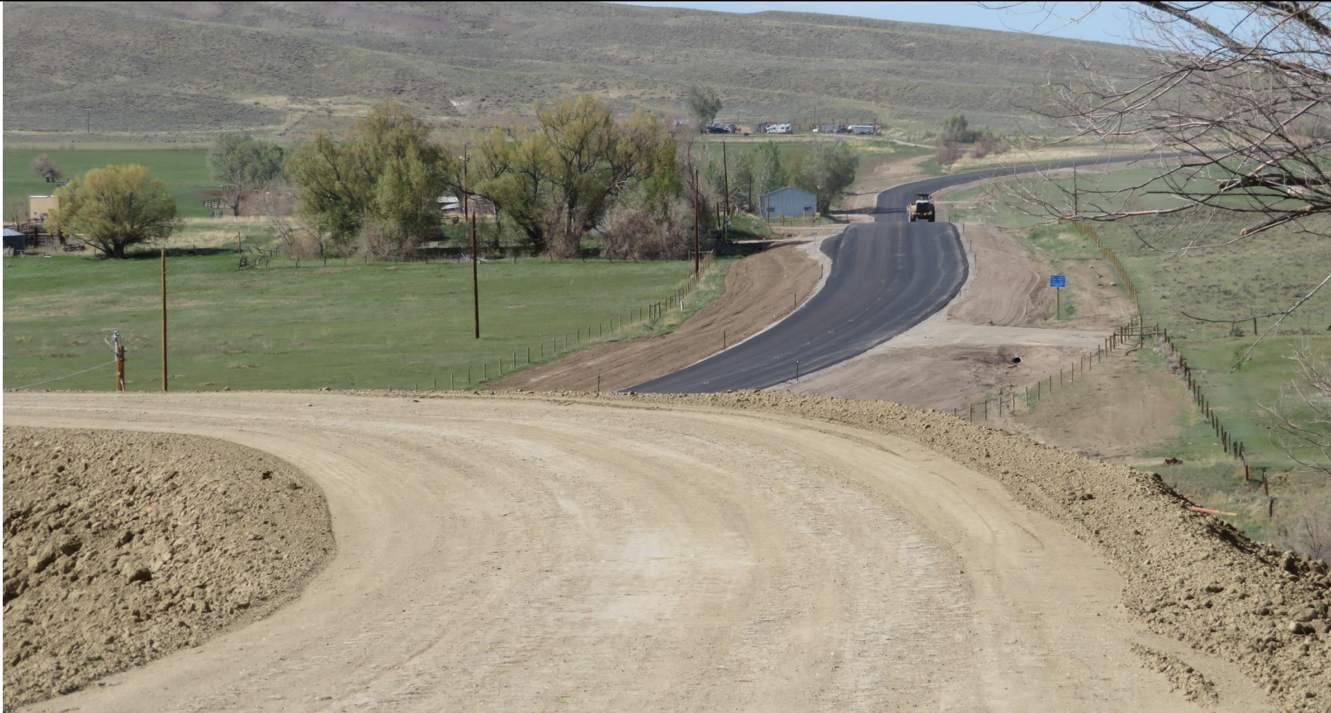
Ethete South (WY132) highway reconstruction
