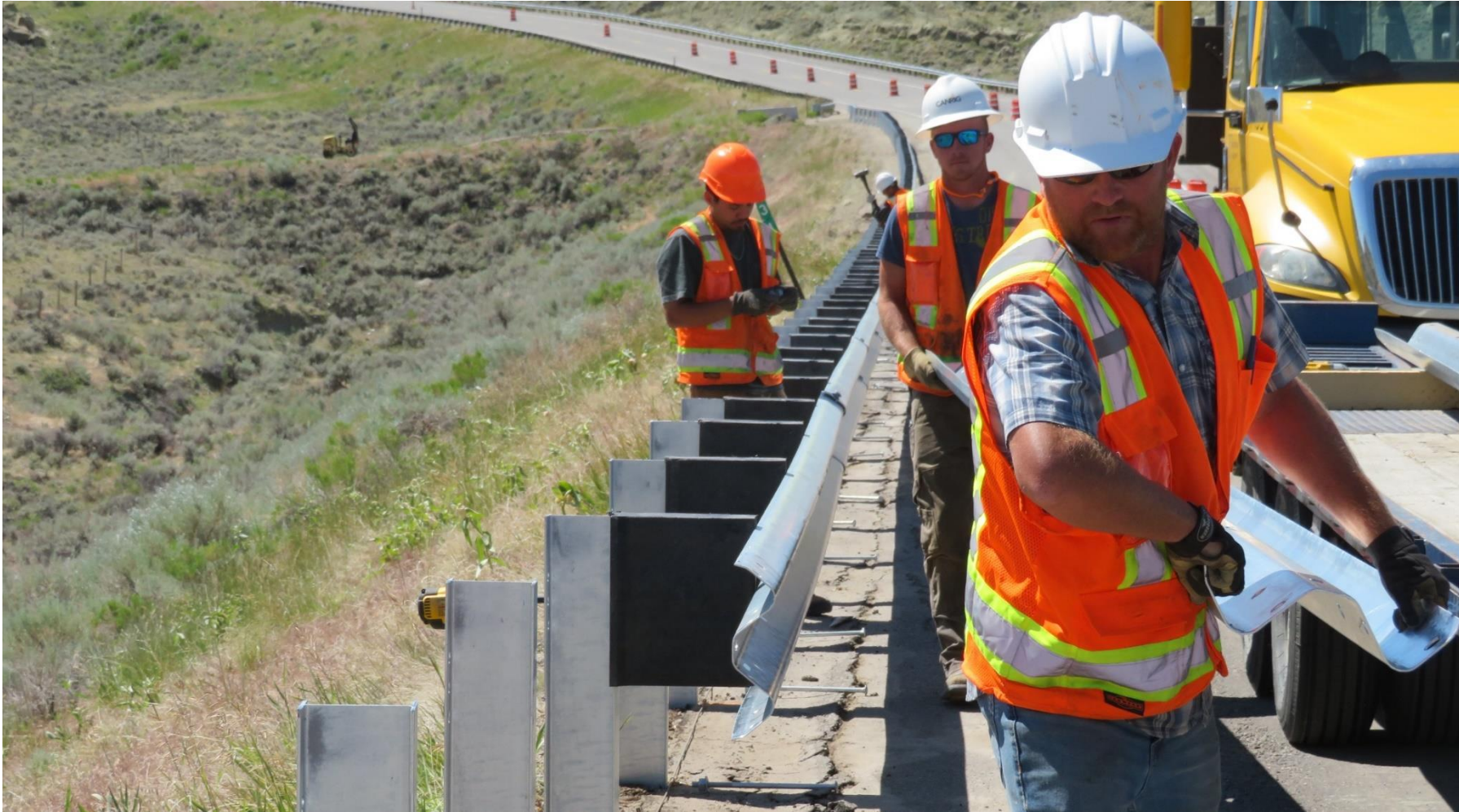
District guardrail upgrade project
