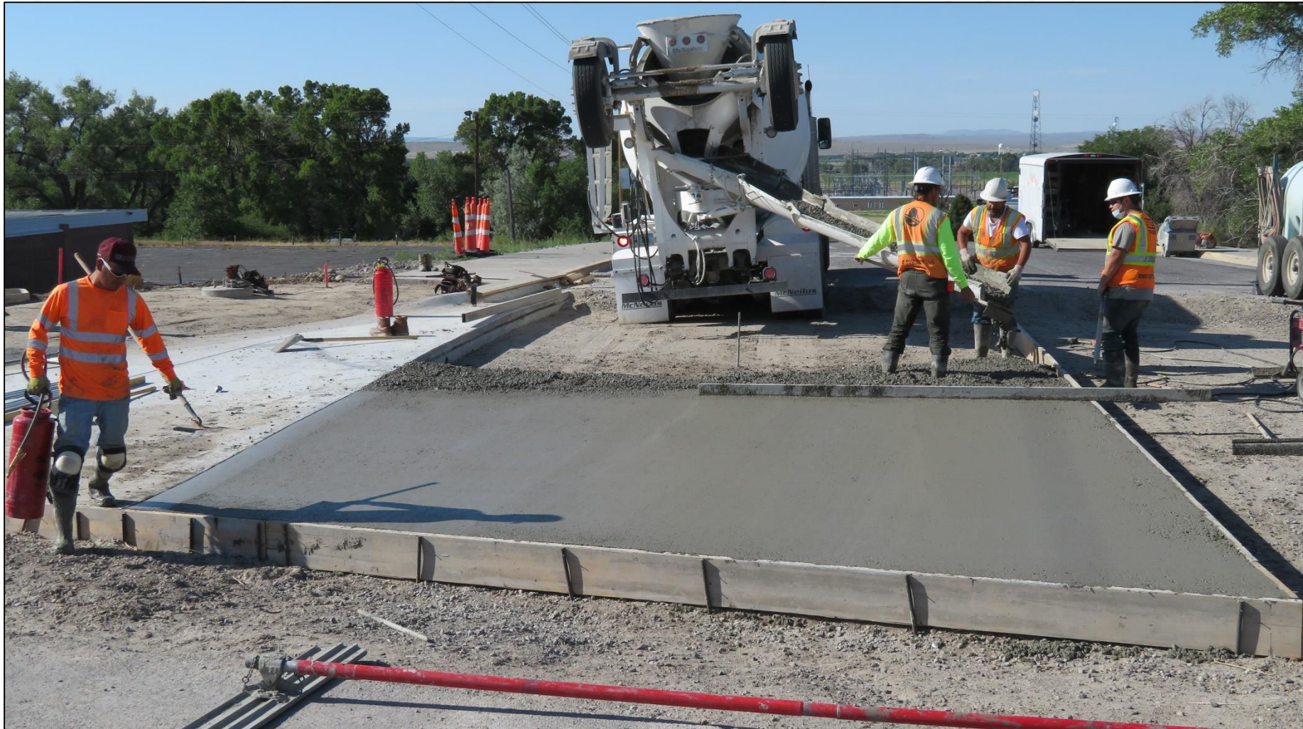
Riverton Main Street ADA/Major Avenue traffic signal
