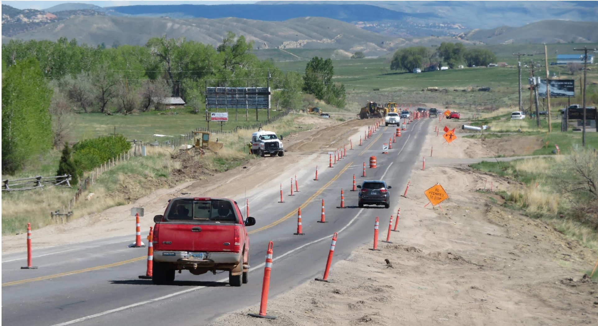
Lander South (US287) roadway widening project
