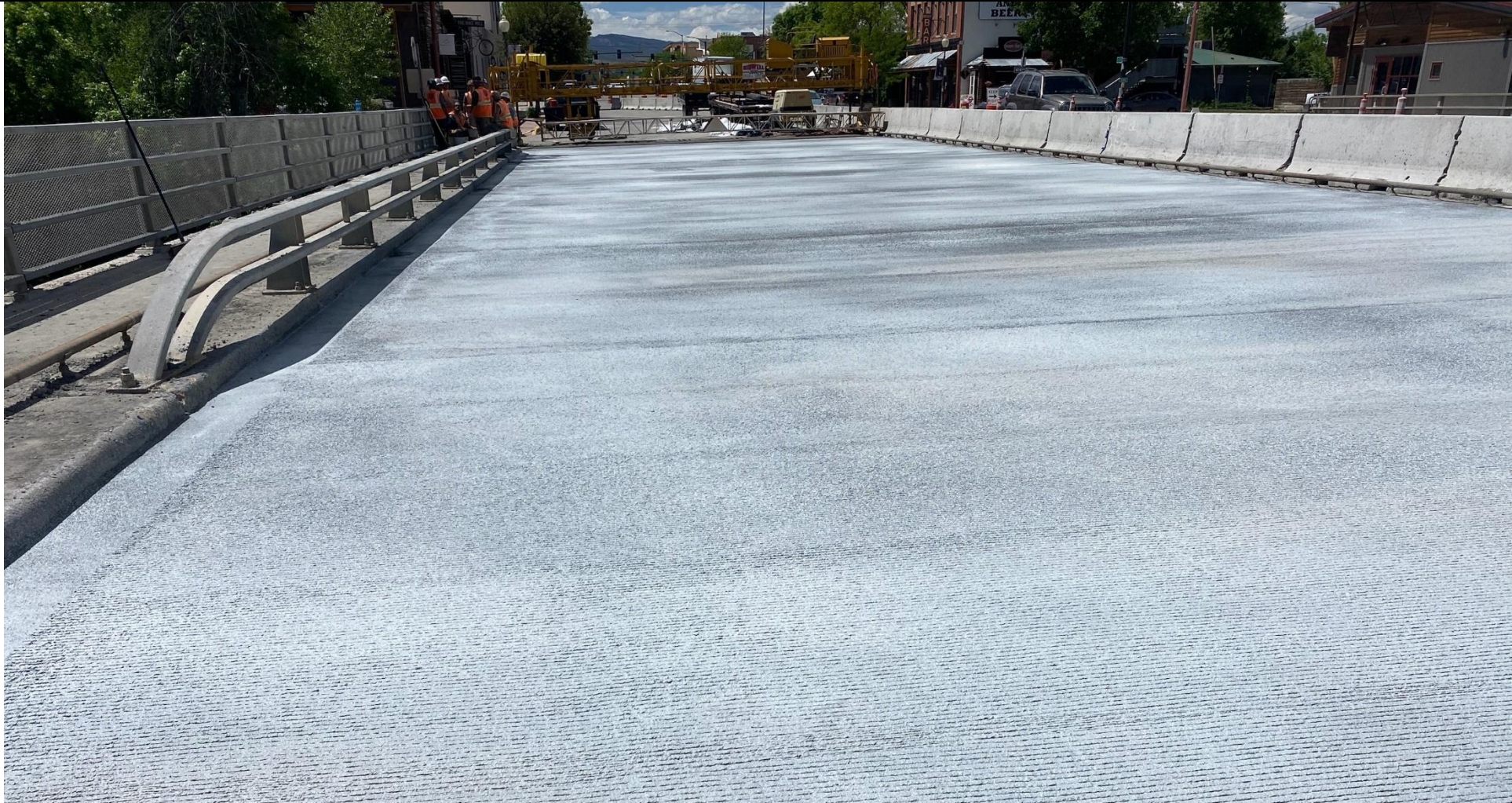
US287/Middle Fork of the Popo Agie bridge rehabilitation
