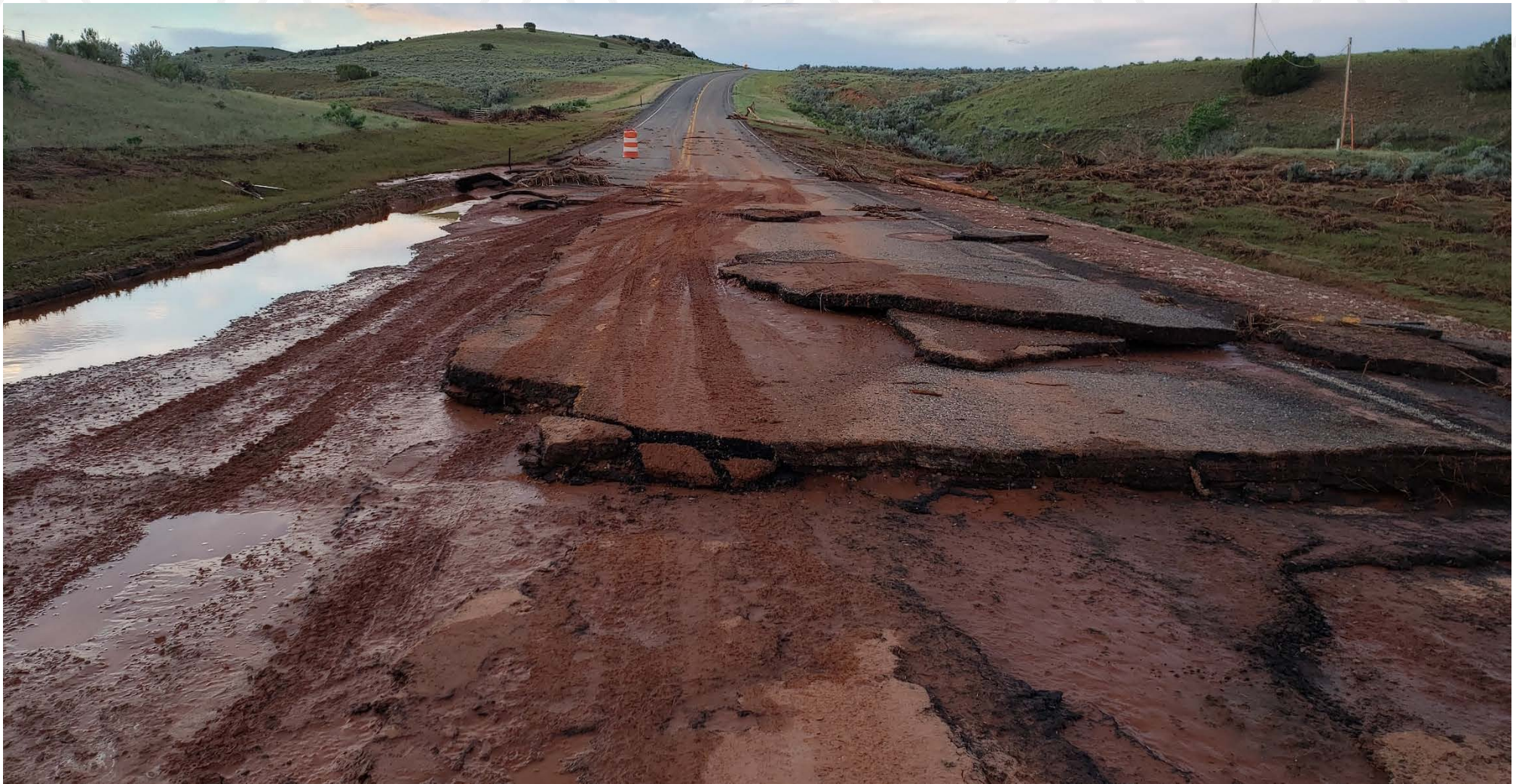
WY434 Big Trails spring flooding damage, Ten Sleep 2020
