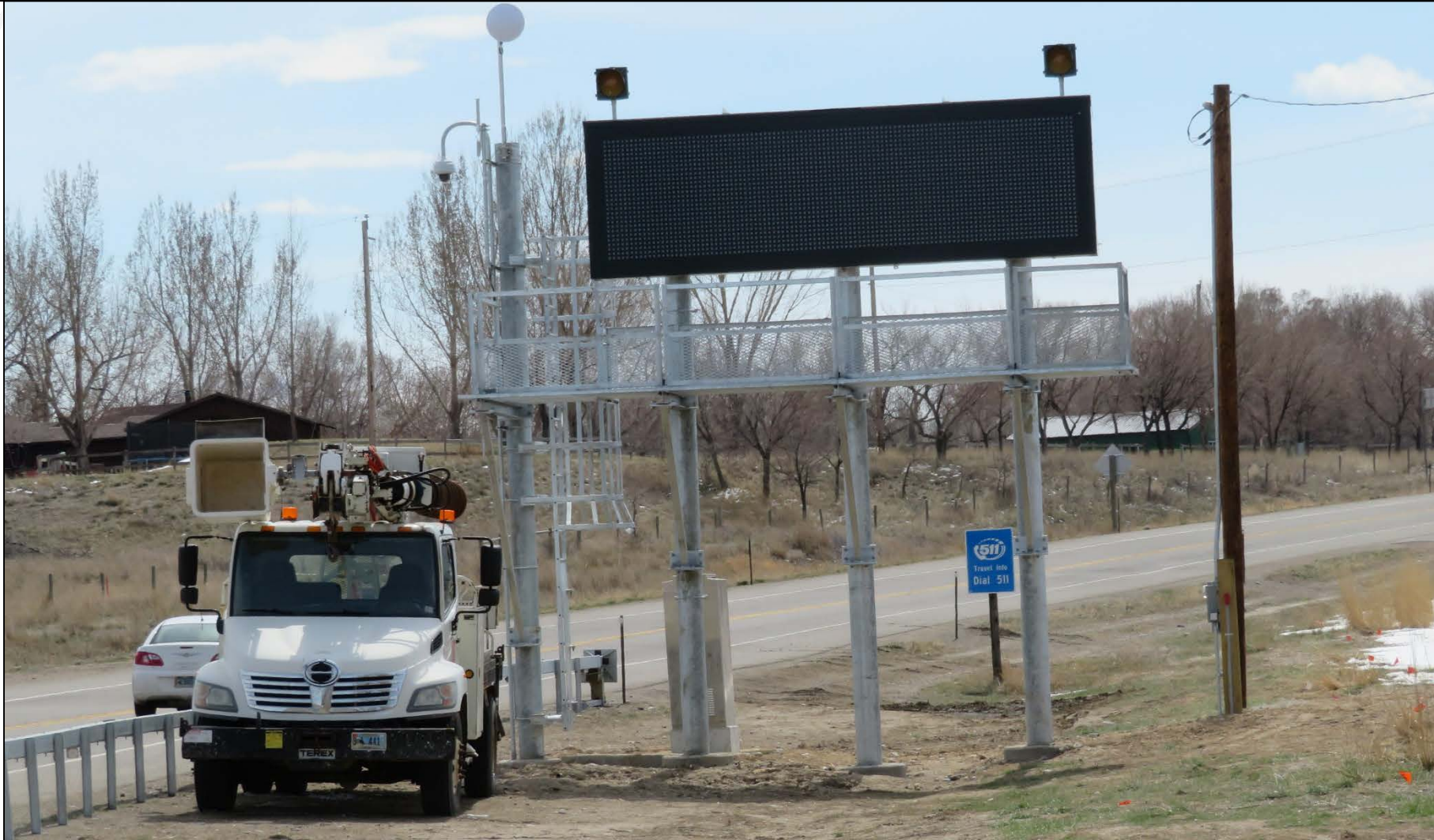
US20 Digital Message Sign installation, Worland, 2020
